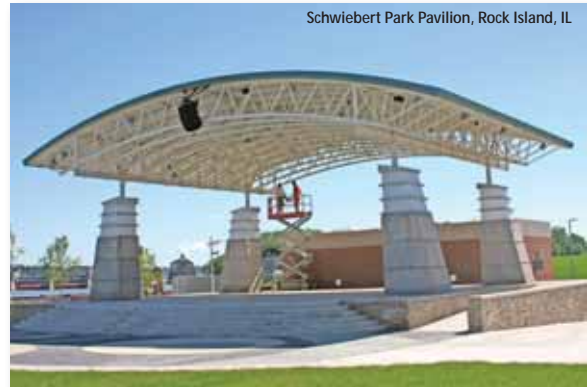
This pavilion's open steel framing offered birds safe harbor. After careful observation and measurement, K-Net was installed with a cable system to keep birds out and surfaces clean.
